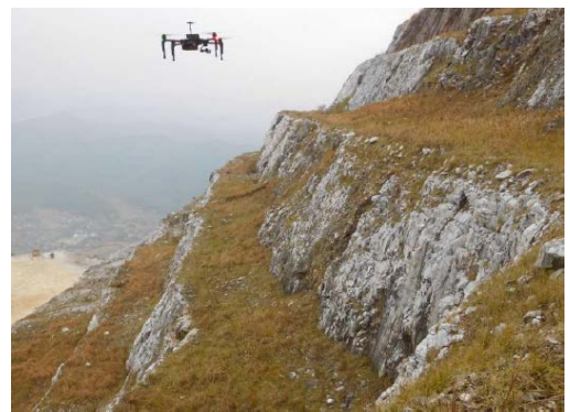
(残壁の浮石点検)
